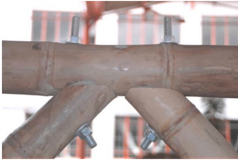
Fig.27. Detail Bonding Anchor Type. Simon Velez 14
