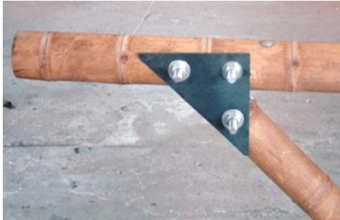
Fig.28. Detail Triangular Plate Type. Simon Velez 14
